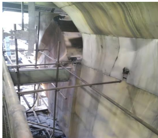
Fig 9. Approach made with scaffolding
