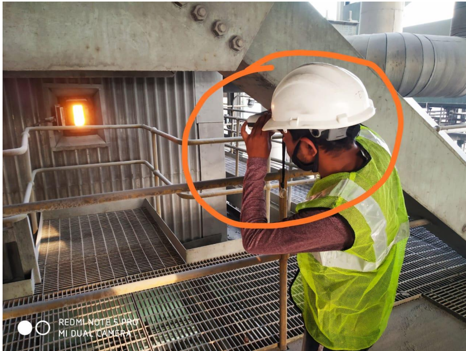
Fig 6. Furnace Temperature Mapping in progress using Infrared Pyrometer
