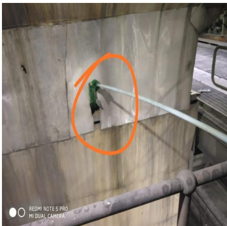
Fig 8. Ingress Point found in checking
