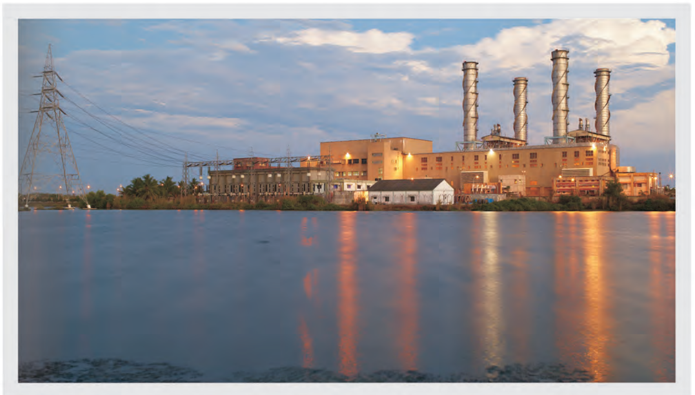
NTPC Kayamkulam Power Station
