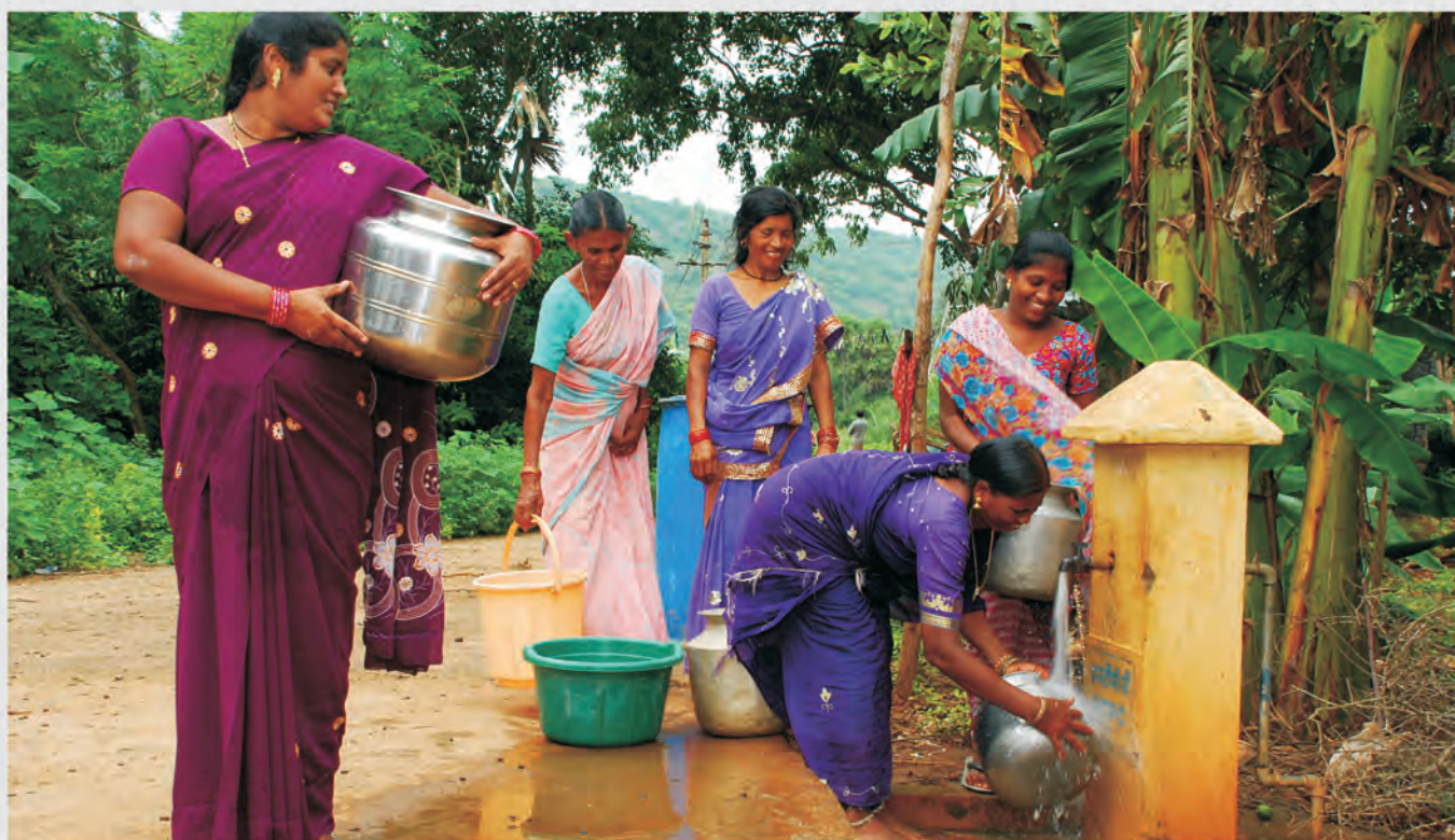
Piped water supply provided by NTPC Ramagundam in nearby village
